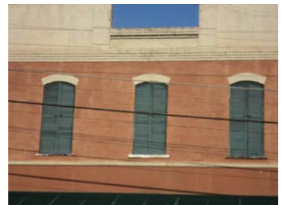
These narrow windows with their arched lintels and painted shutters provide this commercial building with much of its character. The shutters help prevent heat gain from the sun, and protect the windows themselves. Clinton, 2011.
