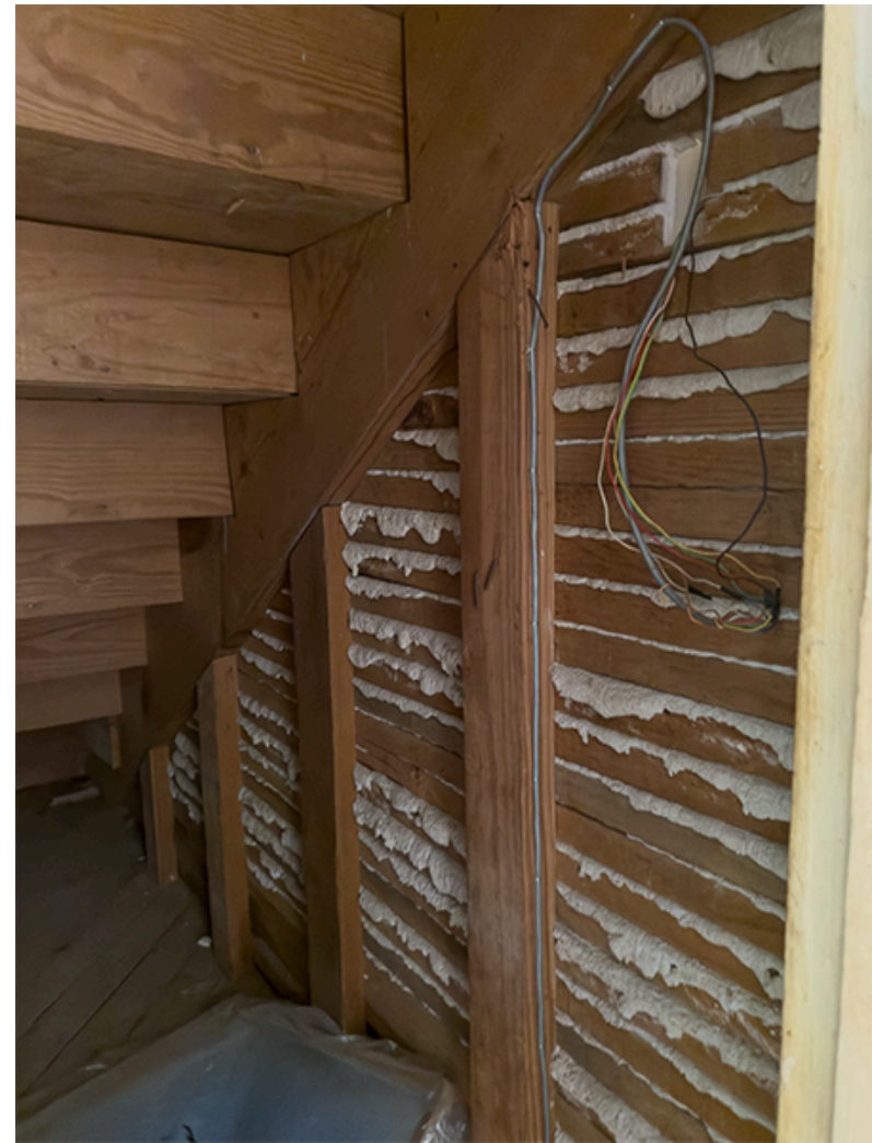
14. Plaster and Lath visible under stairs
