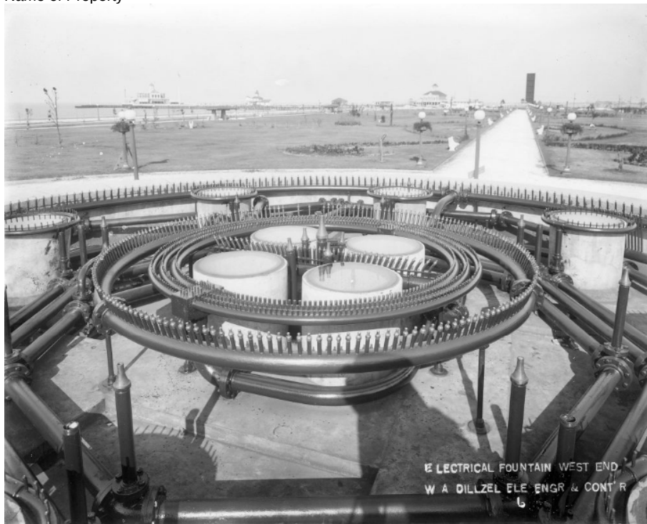
Figure 8: View of the Darlington Electric Prismatic Fountain Heads, Shade Pavilions in Background, 1915 (W.A. Dillzel, City Engineer).
