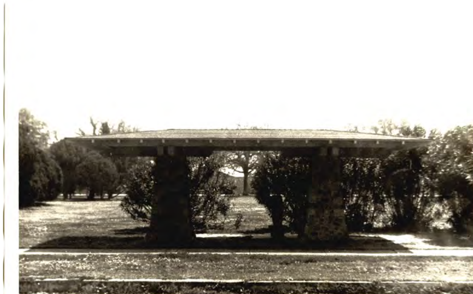
Figure 9: View of a typical Shade Pavilion (New Orleans Public Library).
