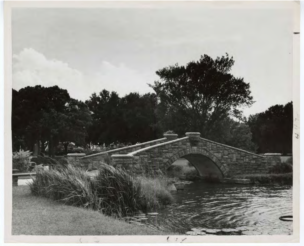
Figure 10: View of the WPA Stone Arch Lagoon Bridge at the eastern end of the park (New Orleans Public Library).
