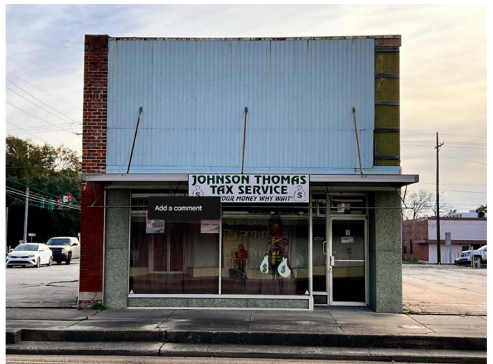
Figure 4. Building located at 110 S. Main Street. Daily World . "Some History of St. Landry Parish from the 1690s on" November 3, 1955.
