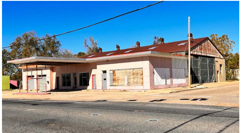
Figure 6. 406 W. Landry Street. Daily World . "Some History of St. Landry Parish from the 1690s on" November 3, 1955.
