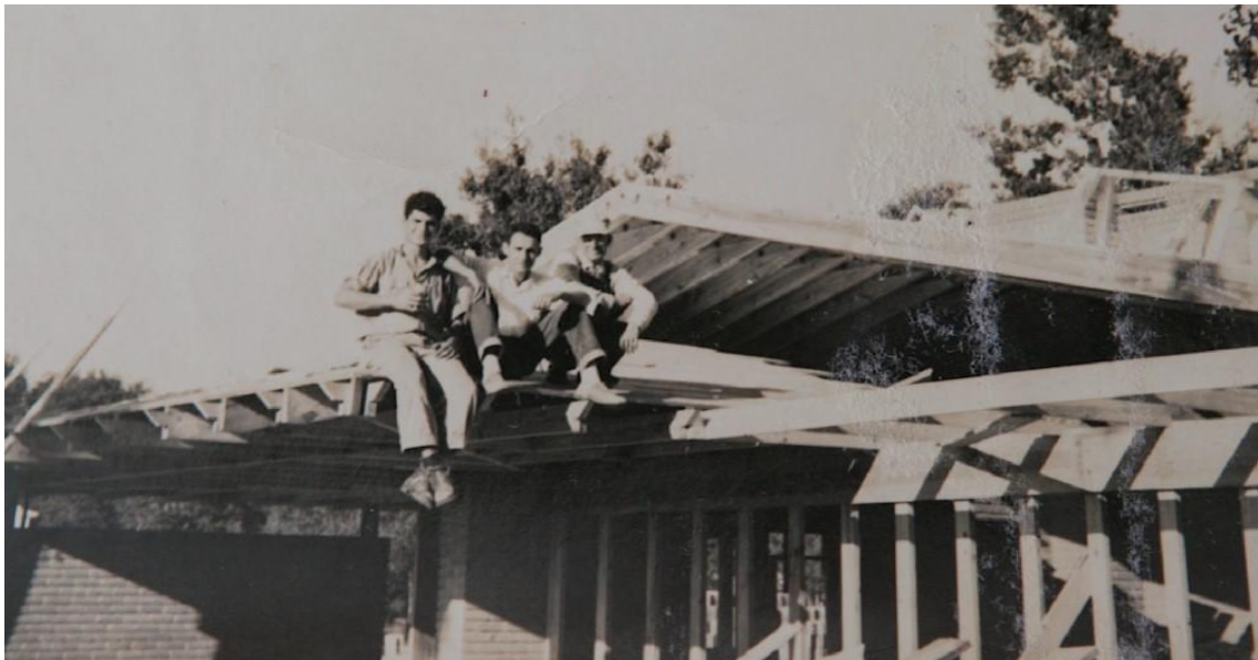
Figure 4. Construction of the Goldate House. Still from Catherine Ledner and Roy R. Beeson. "Designing Life: The Modernist Architecture of Albert C. Ledner." Short film. Release August 25, 2017.
