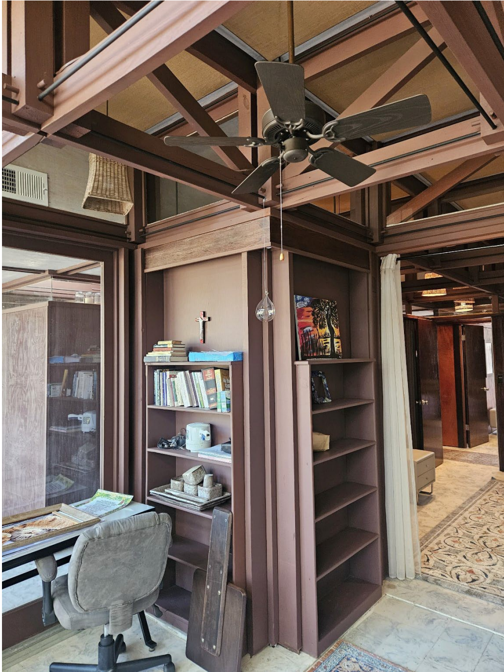
Photo # 14. General view showing one of 4 structural cores that supports the space frame roof, which is functional used as a closet, in the sitting room off of the bedroom in the north corner of the building, looking south.
