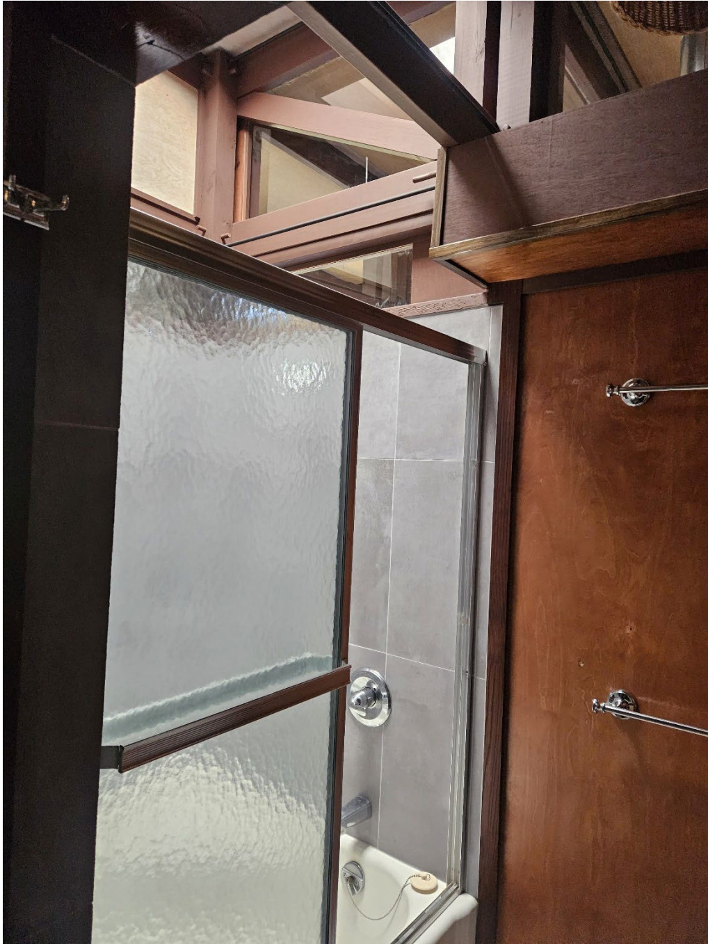
Photo # 15. General view showing the historic bathroom on the northwest side of the building, looking north.
