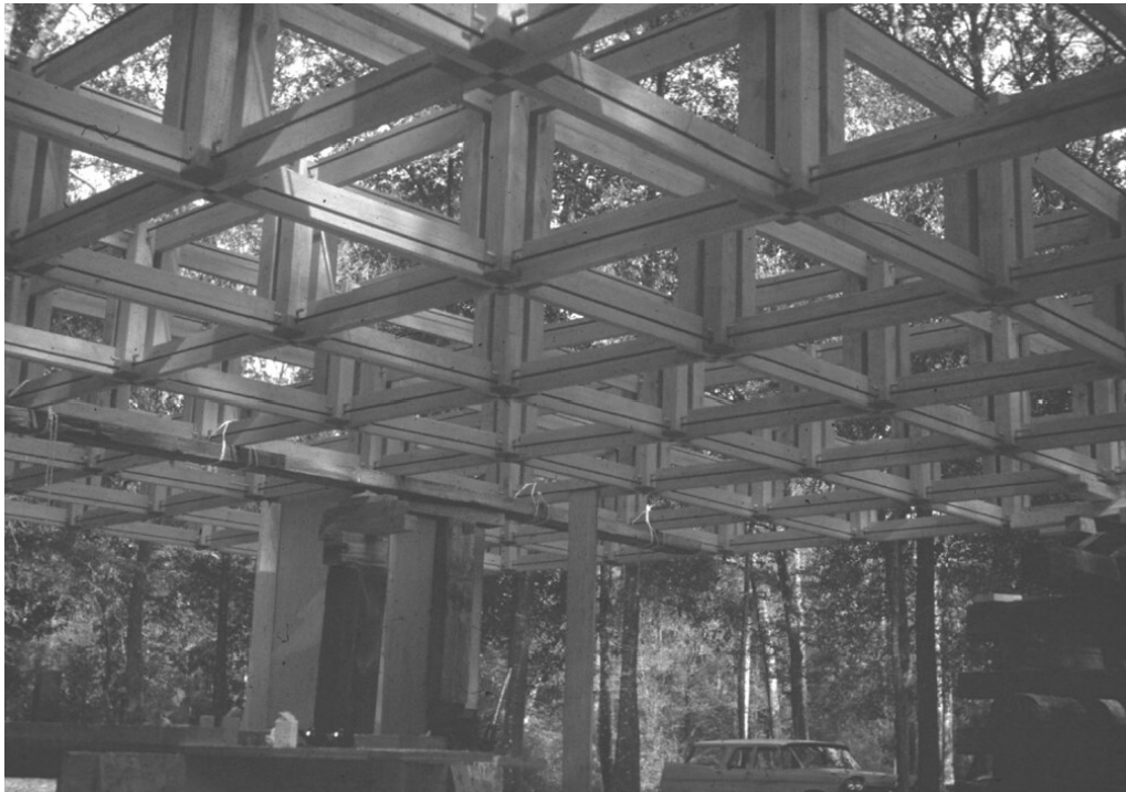
Figure 3. The Mollere House's "space frame" roof under construction, 1959, Tulane University Special Collections
