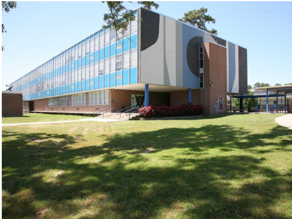
Figure 23. Woodlawn High School, 7340 Wyngate Boulevard, Shreveport, LA. Unexpected Modernism, The Wiener Brothers Story. UnexpectedModernism.com.
