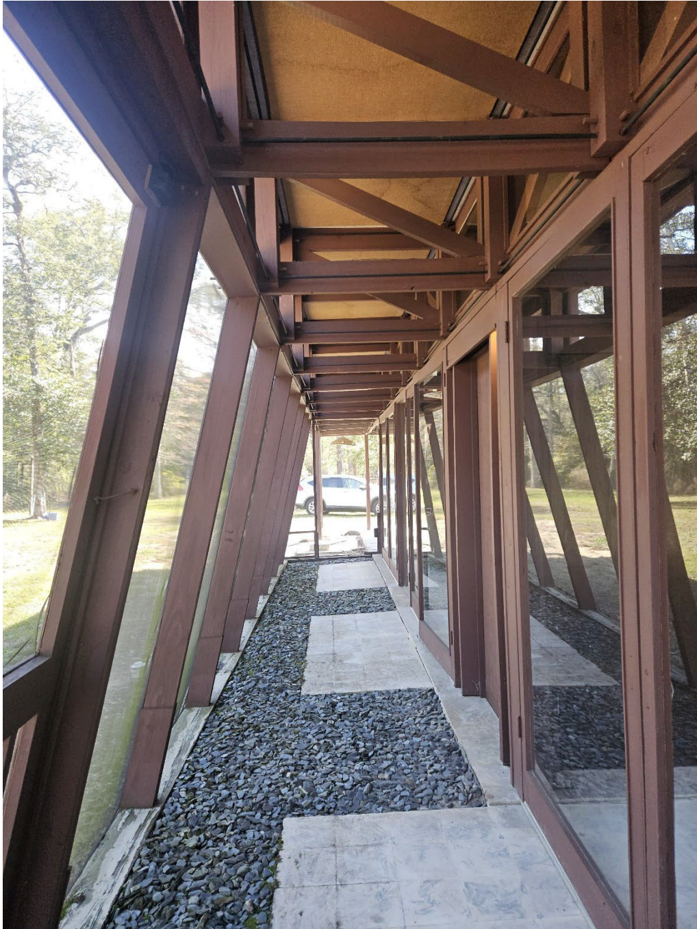
Photo # 18. General view showing an exterior screened corridor on the northeast side of the building, looking southeast.
