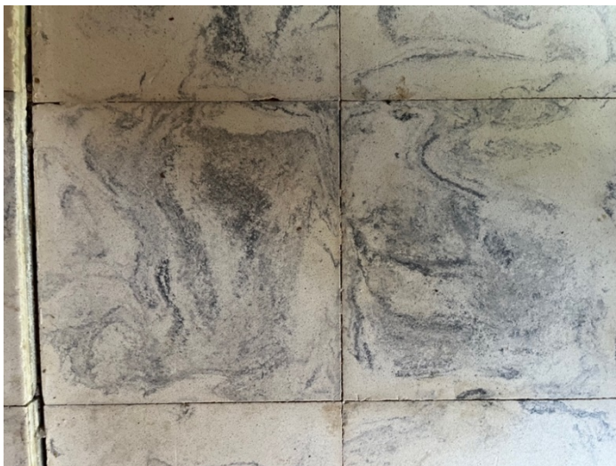
Figure 2. White pre-cast concrete floor tiles with light grey-blue designs, meant to mimic marble.
