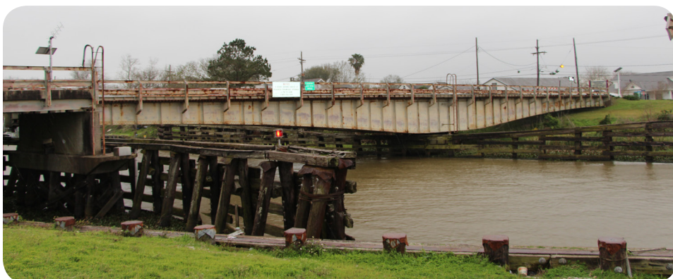
This 1940 swing bridge features what is known as a bobtail swing span due to span arms that are different lengths on either side of the pivot pier (Bayou Lafourche-Lockport Bridge, Bridge Recall No. 001304).
