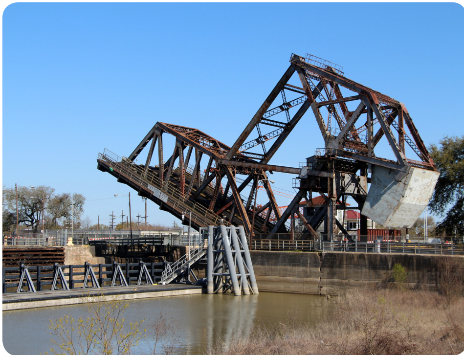
This 1919 Strauss heel trunnion bascule bridge was a boon to transportation since it served rail and vehicular traffic (St. Claude Avenue Bridge, Bridge Recall No. 001570).
