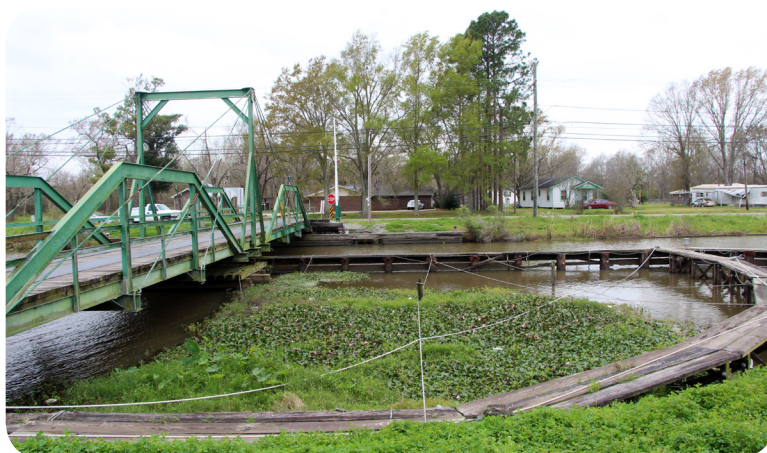
Cable-stayed swing bridge with its characteristic system of ropes and pulleys that operate the bridge (Terrebonne Parish Road No. 293 Bridge, Bridge Recall No. 200852).
