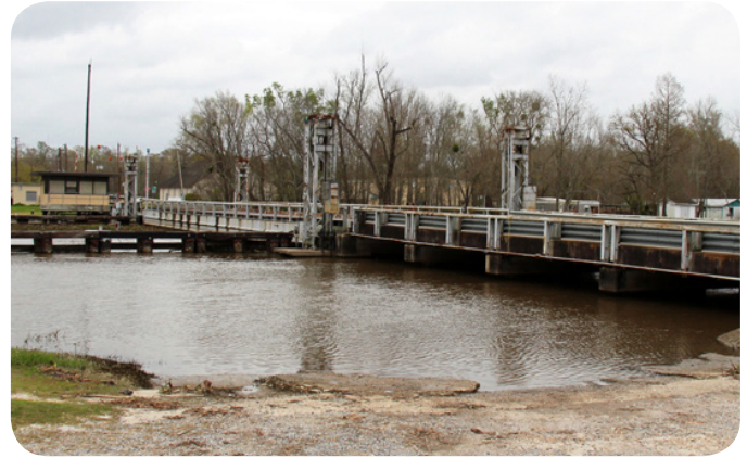
Pontoon swing bridge in the closed position (Lower Grand River Bridge, Bridge Recall No. 054480).
