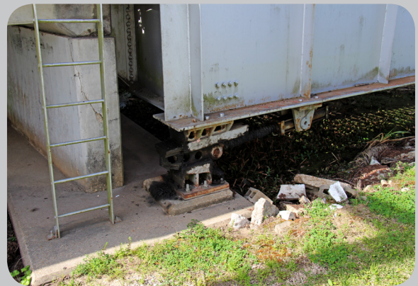
Wedge drive with hydraulic cylinder (Bayou Pierre Part Bridge, Bridge Recall No. 051500).
