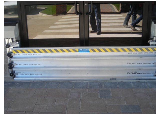
Stackable flood barriers deployed at entrance (2011)
