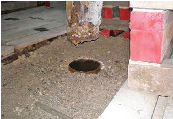
Disconnection of Pipe
