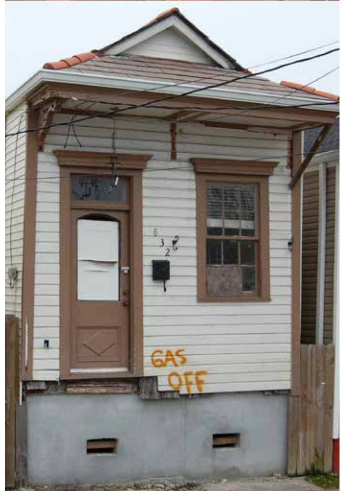
Top Left: House in New Orleans that was elevated after Hurricane Katrina.
