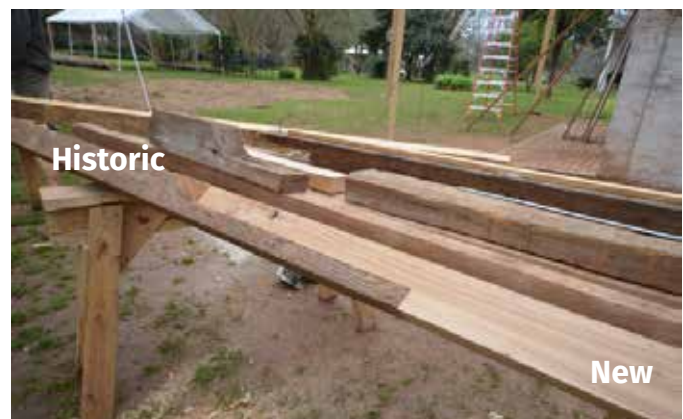
This historic cypress rafter has a new cypress piece sistered in to replace damaged material. The darker wood is the historic material that was retained. Image Credit: NPS|Sarah Marie Jackson.
